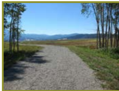
Newly constructed elevated trail near Henry Road by Nicki Feiten
